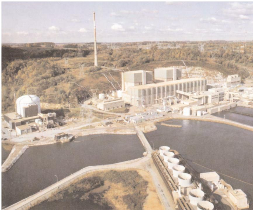
*Peach Bottom Unit 1 (far left), in York County, Pennsylvania, was a 40-megawatt experimental high-temperature, helium-cooled reactor that gave the United States experience with this type of reactor, during its 1967-1974 operation.*
